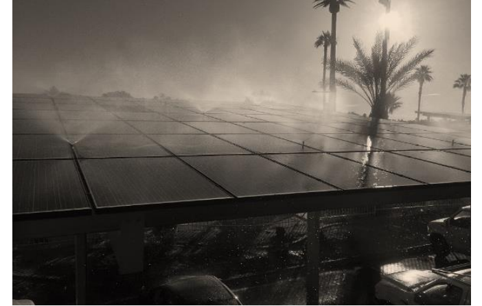
Manual wiping with automatic nozzles
